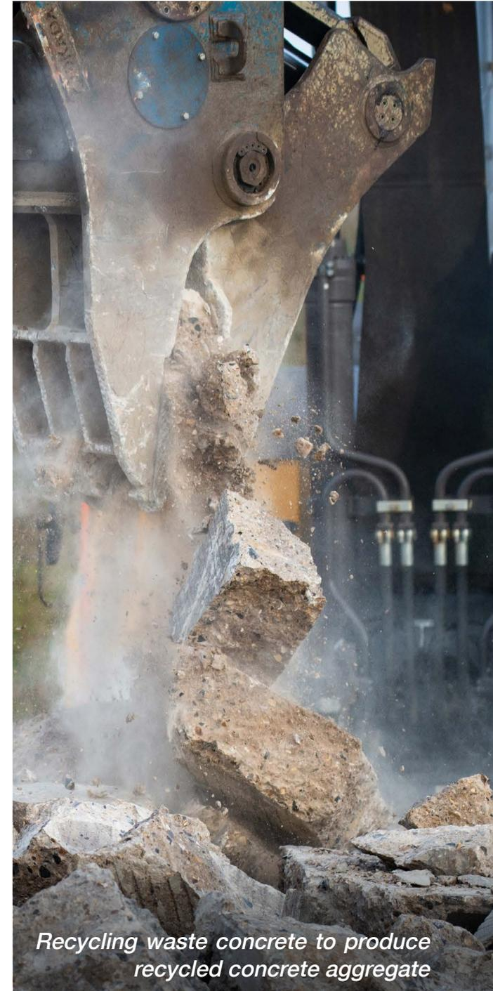
*Recycling waste concrete to produce recycled concrete aggregate*
