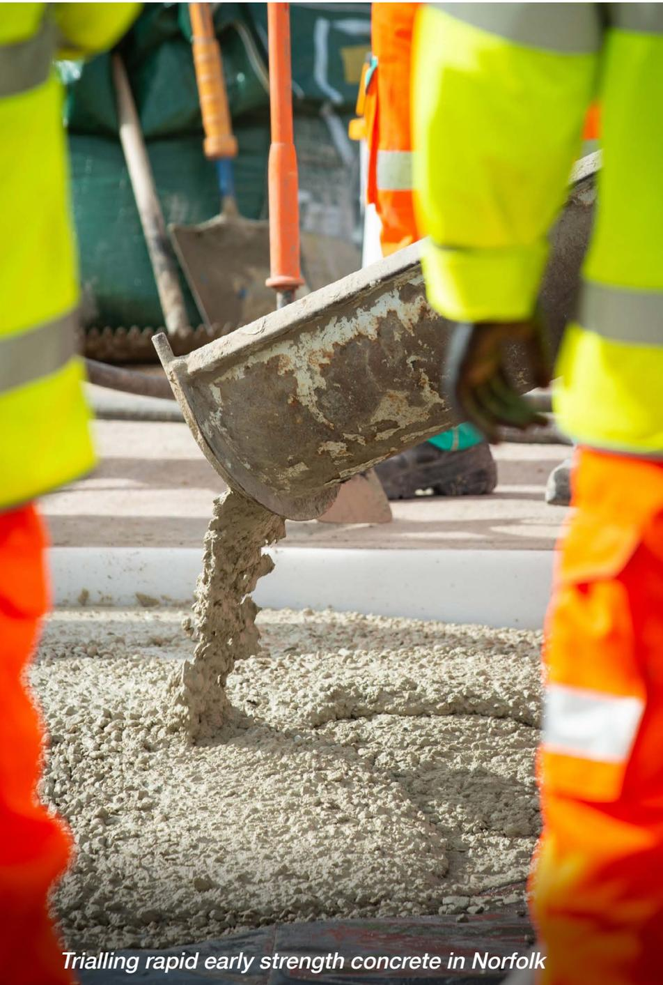
*Trialling rapid early strength concrete in Norfolk*
