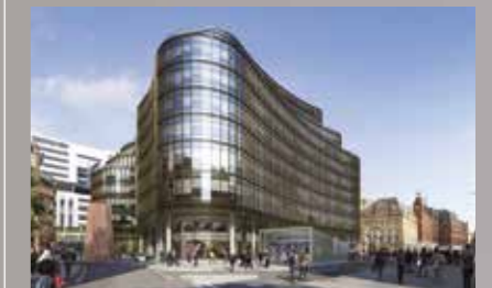
SMBC 100 Liverpool Street, EC2 161,000 sq ft, under construction
