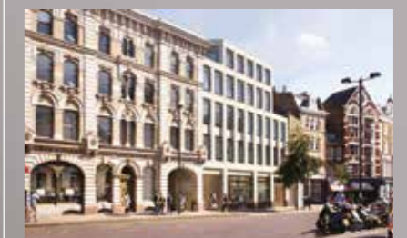
LiveNation Farmiloe Building, 34 St John Street, EC1 63,000 sq ft, under construction
